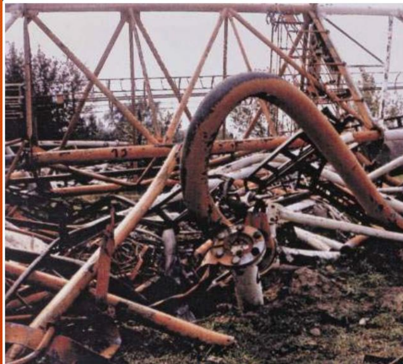
Fig. 1: The tallest mast in the World, the 648 m high long wave mast in Konstantynow, Poland collapsed in 1991
