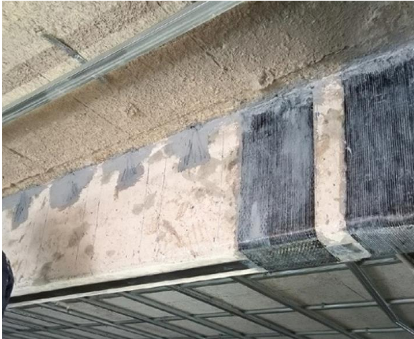
Anchorage of U-shaped FRP wraps using FRP strings.
