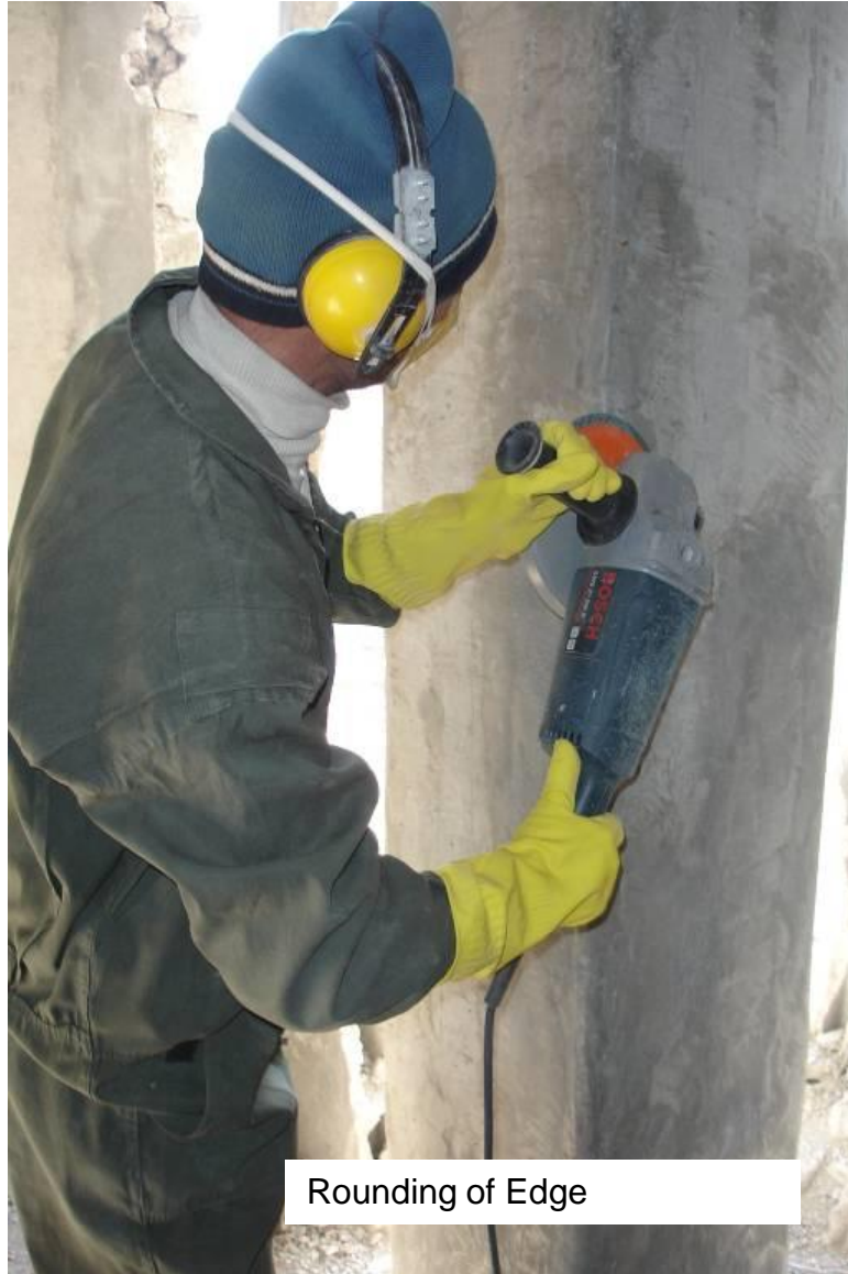
preparation of the substrate
